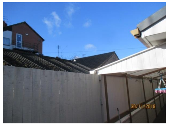
Boundary between site and 2 Lily Grove (looking towards 2A Lily Grove)
